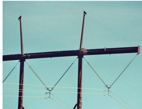
Common raven nest on transmission pole with steel "Y" discouragers.
