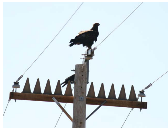
Golden eagle perched on distribution pole with cone discouragers, and common raven perched on conductor
