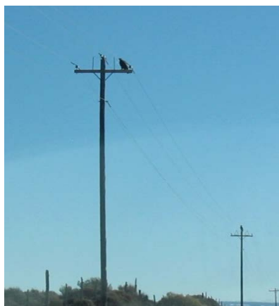
Golden eagles perched on adjacent distribution poles with moving/hazing and barrier-type discouragers
