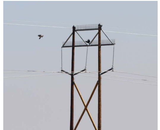
Red-tailed hawk (left) flushing common raven (right) from transmission pole with perch discouragers.
